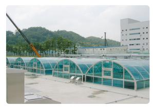
Dome type waste water purification control unit to prevent the odor scattering (Tangjeong Plant)
