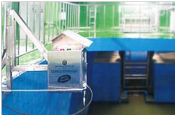
Oil/Water Separation Facility
