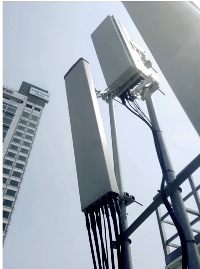
Figure 4: Co-located 32T32R and 8T8R MIMO antennas
