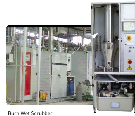
Burn Wet Scrubber
