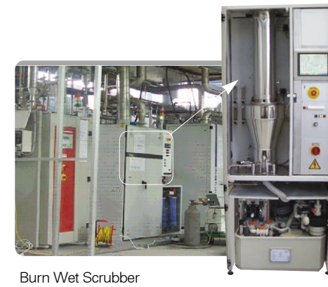
Burn Wet Scrubber
