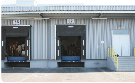
SHUTTER at receiving and shipping dock
