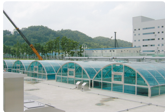
Dome type waste water purification control unit to prevent the odor scattering (Tangjeong Plant)
