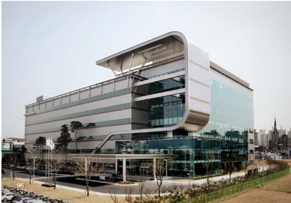
ICT Suwon Center (Green Data Center)
