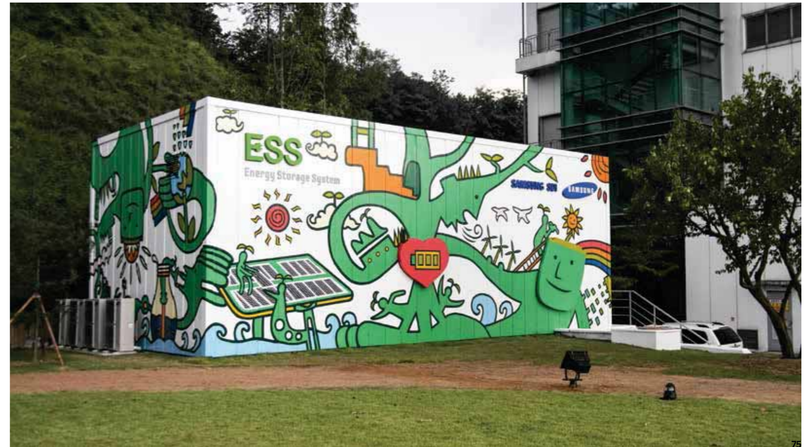
Energy Storage System (ESS)
