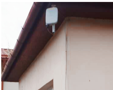
Figure 15 : Outdoor CPE installed in the residence of a friendly user
