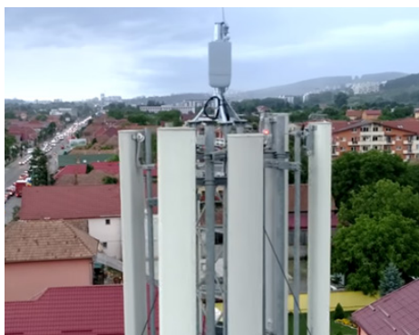
Figure 13 : Cell15 Rooftop and AU Location
