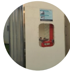
Outdoor emergency washing facility
