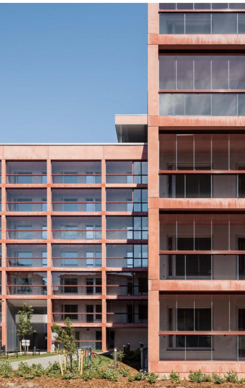
fot. Maxime Verret; Trévoux 84 Housing Units, Tectoniques
