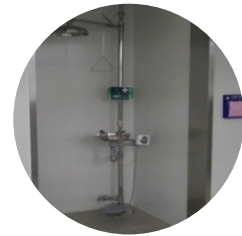
Indoor emergency washing facility
