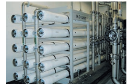
Industrial water treatment system
