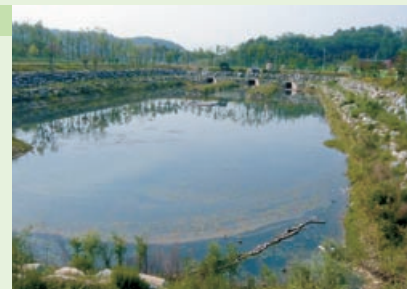
Tangjeong Factory detention pond
