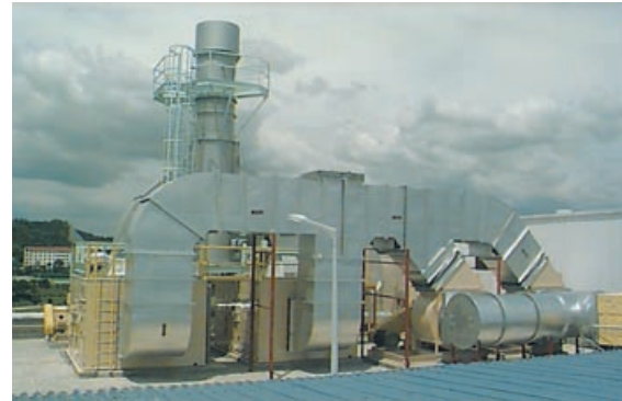
VOC treatment facility
