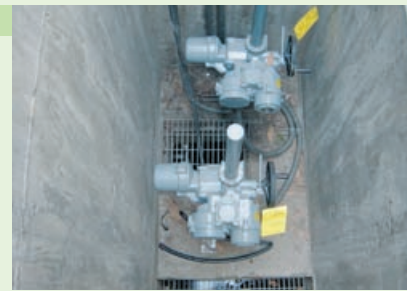
Oil/water separation system
