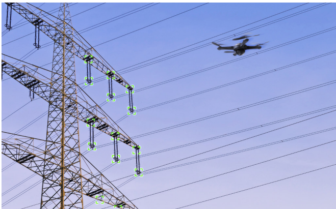
Figure 10: Thermal Camera Attached Drone Taking Photos to Check the Grid Status
