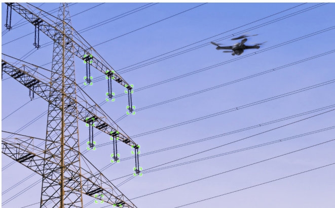
Figure 10: Thermal Camera Attached Drone Taking Photos to Check the Grid Status
